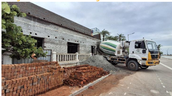
Figure 53: Pudumai building under Construction
