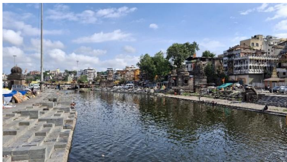
Figure 44: Goda Ghat Steps constructed under SCM
