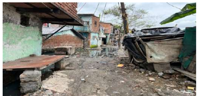
The streets are lower than the Taimoor Nagar Drain flooded with back flows from the drain.
