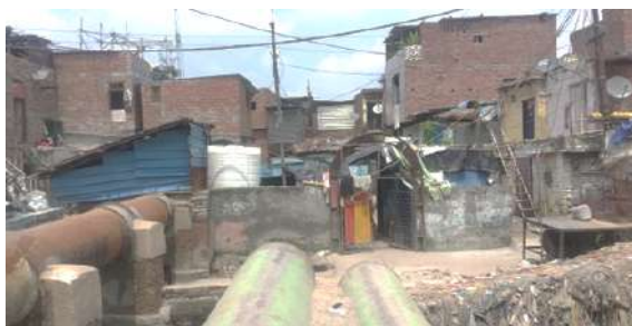
Entrance of the Community as well as the Community toilet is shown in the red circle
