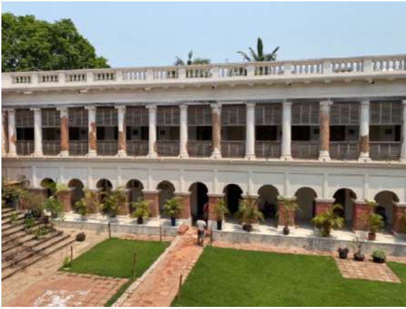
Figure 11. Bawali Rajbari East Wing post restoration
